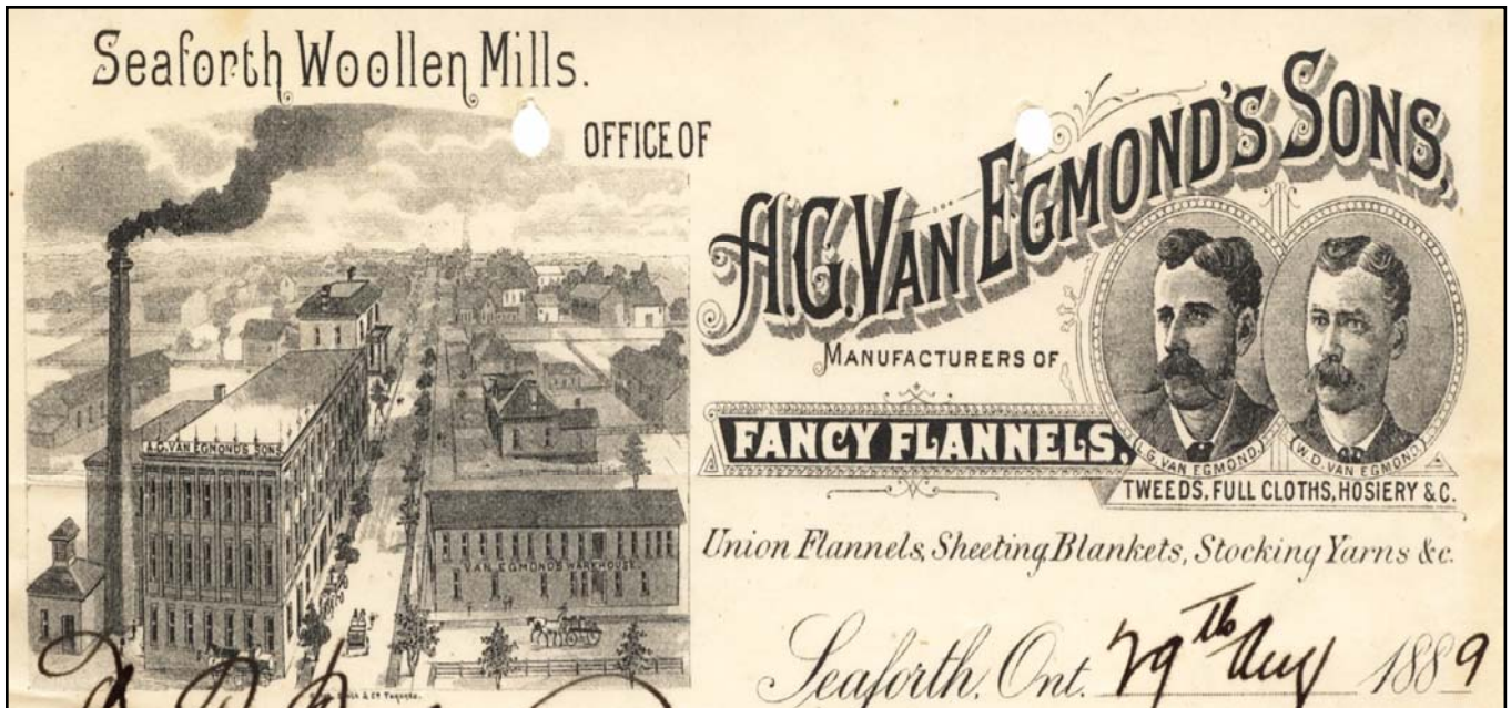
Shown at the right of this receipt dated August 29 th , 1889 are Leopold G. and William D. Van Egmond. The mill building, built in 1884, had 27 lightning rods. The mill's whistle when blown made three different sounds at the same time.
