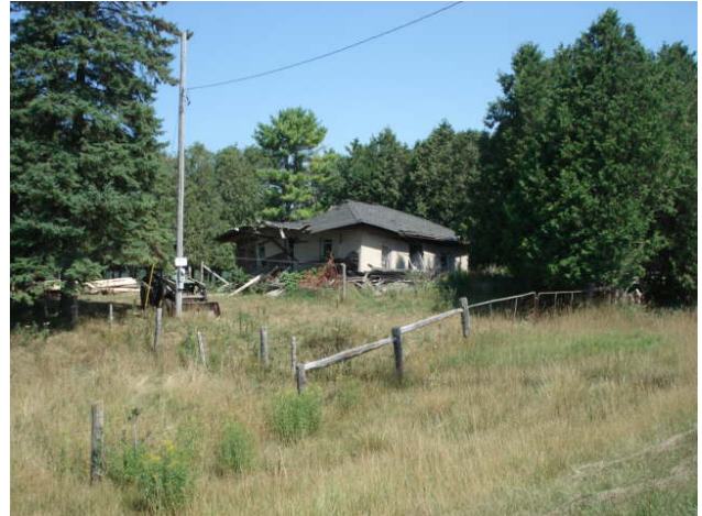
Continuing structural distress through 2006
