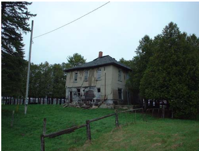
Started to "bulge" in May, 2004
